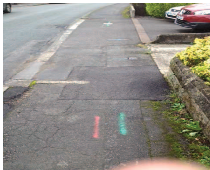
Photos showing condition 3 footway – Functionally Impaired
