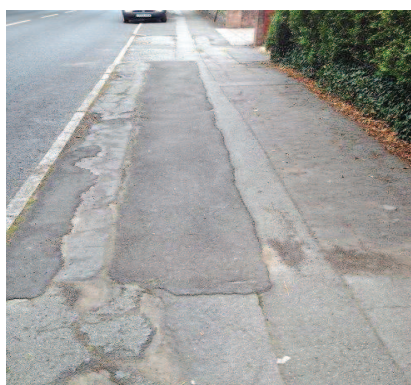
Photos showing condition 4 footway – Structurally unsound
