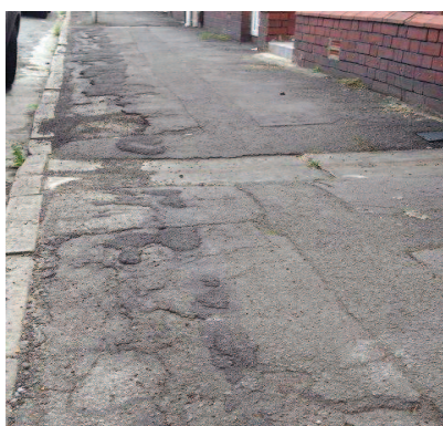
Photos showing condition 4 footway – Structurally unsound
