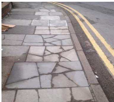
Photos showing condition 3 footway – Functionally Impaired
