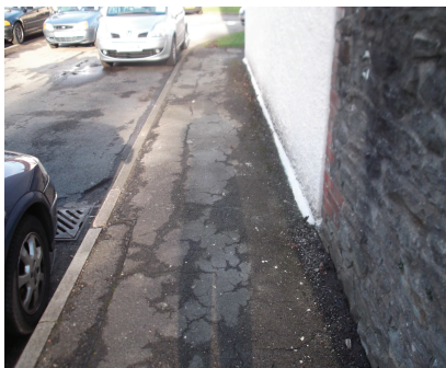
Photos showing condition 2 footway – Aesthetically Impaired
