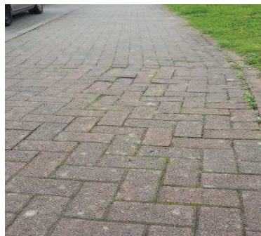
Photos showing condition 2 footway – Aesthetically Impaired
